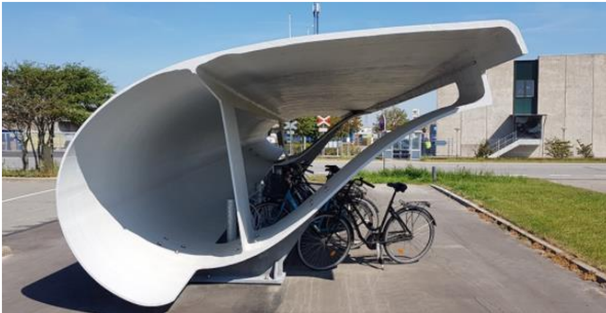
Figure 3-6: Innovative use of repurposed wind turbine blade to provide secure sheltered landmark bicycle parking
